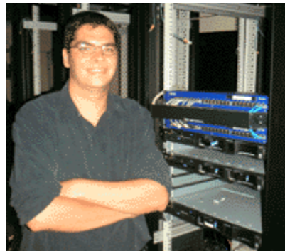
AT&T's Fred Chagnon with rack mounted Perle Console Servers
