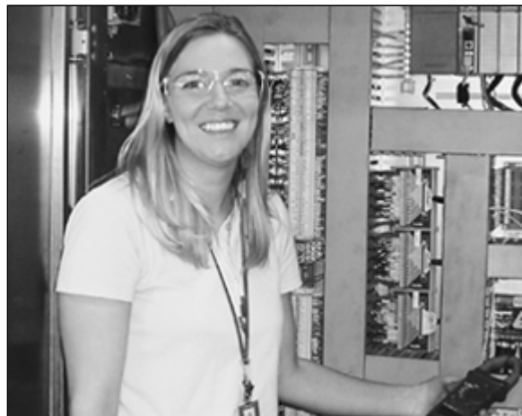
At Energizer, electrical engineer Tara Kohmetscher installs battery manufacturing equipment.
